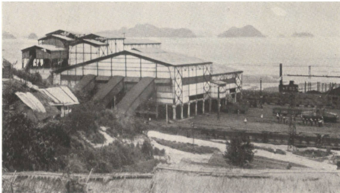
Screening Plant, Campha
