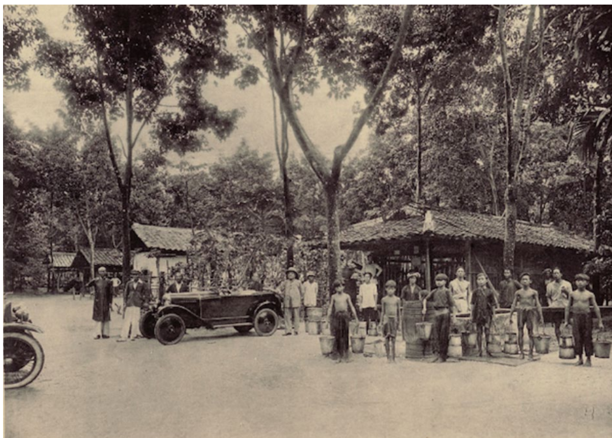
Planche 102. — Usine, atelier, fumoir, hangars
